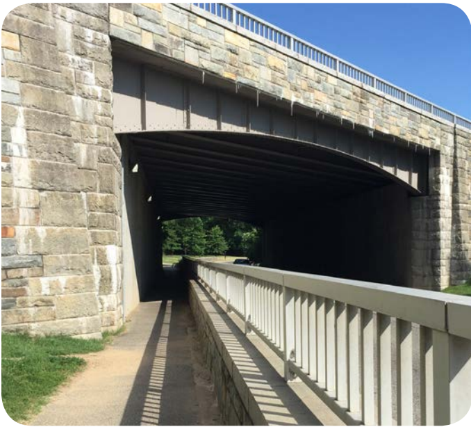
Figure 26 Narrow section of Mount Vernon Trail under the Parkway.
