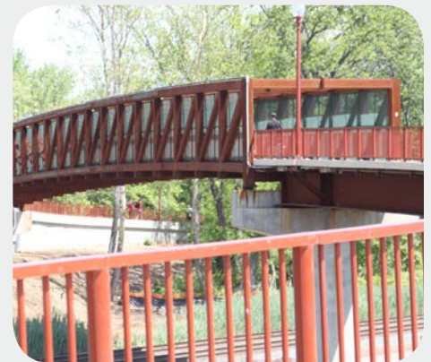
Anacostia Riverwalk Trail Bridge. (DDOT)
