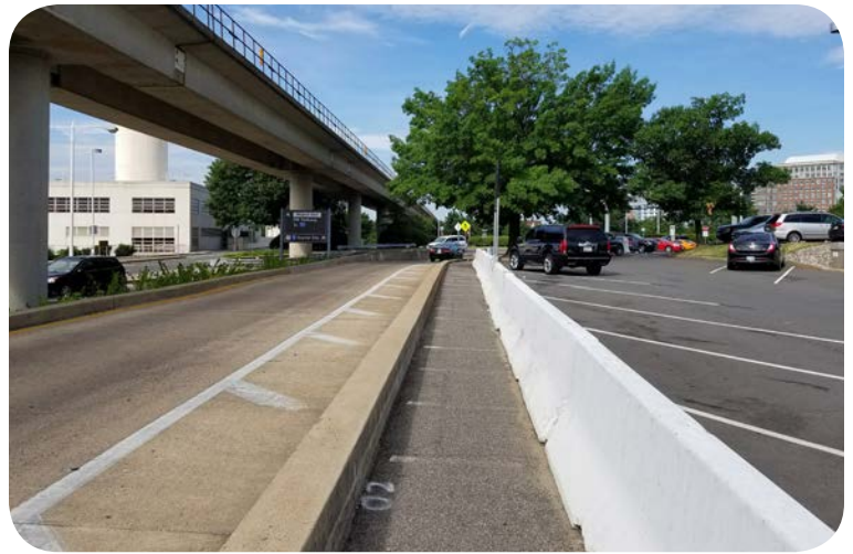
Figure 23 Asphalt sidewalk along Aviation Circle, leading to the 26th Street Bridge Connection from Terminal A.
