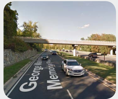
Mount Vernon Trail Overpass near Roosevelt Island. (Google Maps)
