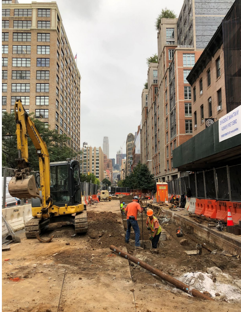
Block by block phased construction mitigated community impacts
